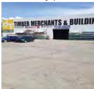
View of: Brick warehouse Looking south Inspected on 25-27.9.2013
