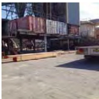
View of: Timber dressing machinery Looking south west Inspected on 25-27.09.2013
